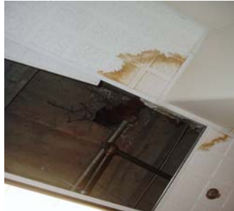
Damaged Ceiling by Water Leak from Roof
