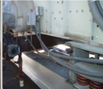
Rusted Cooling Tower Frame & Piping
